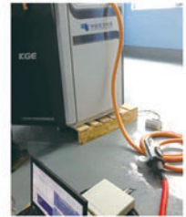
▲ Charging pile troubleshooting for China Southern Power Grid
