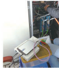
▲ Baiyun Airport Weather Radar Troubleshooting
